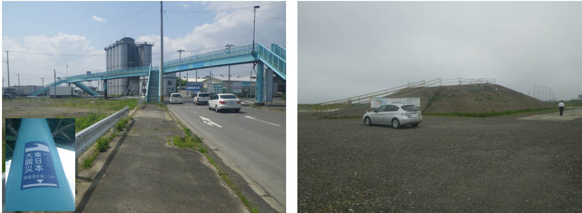
Figure 24 Left: Tsunami inundation mark on the pedestrian bridge that saved many lives in Yuriage (30/5/2012); Right: About 3 m land elevation in Yuriage will be increased as shown in the model
