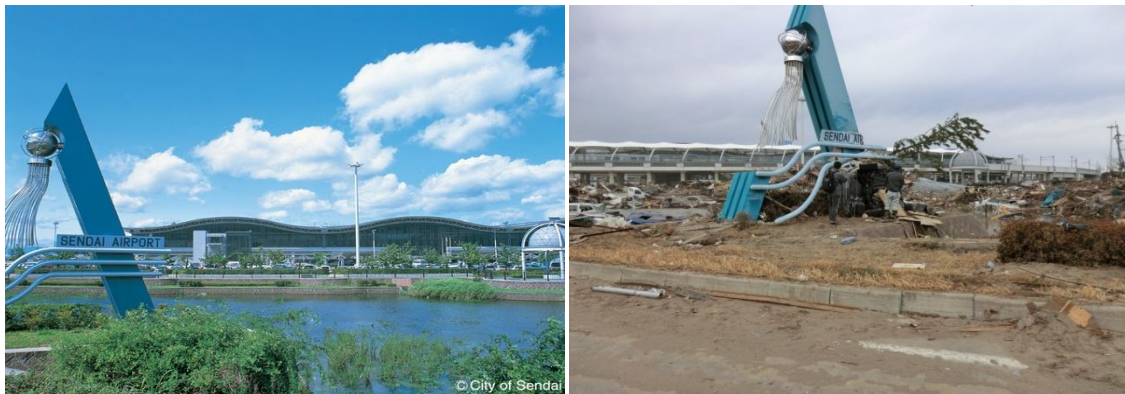
Figure 25 Damages to Sendai Airport ( Left: before [ www.japan-i.jp ]; Right: after)
