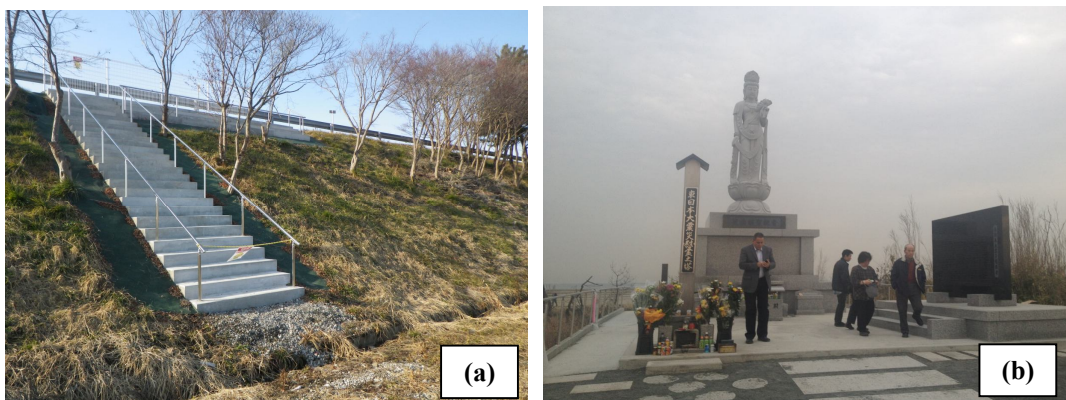
Figure 17 (a) Staircase built for access to the surface of the Sendai-East expressway and (b) New tsunami memorial (13/3/2013)
