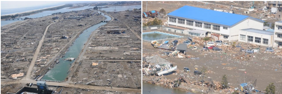
Figure 23 Left: An aerial view of Yuriage in the direction from north to south. The floodgate at the bottom in the photo is the entry point from Natori river to the Teizan Canal. Many bodies and vehicles lie at the bottom of water in this area. Rescue divers have been in search and rescue work since March 19. Right: Yuriage Junior High School served as a temporary evacuation center. Many cars and fishing boats were swept into the school yard. ( Self Defense Force )
